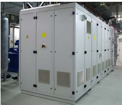
Compressed air reservoir Mixer + Hydraulic supply unit
